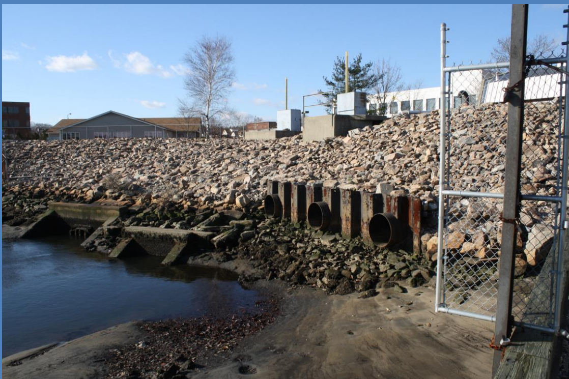
City of New London, Hurricane Barrier at extreme low tide. Note 2 Gravity discharges with tide gates (l), and 3 storm water pump station discharges (r)
