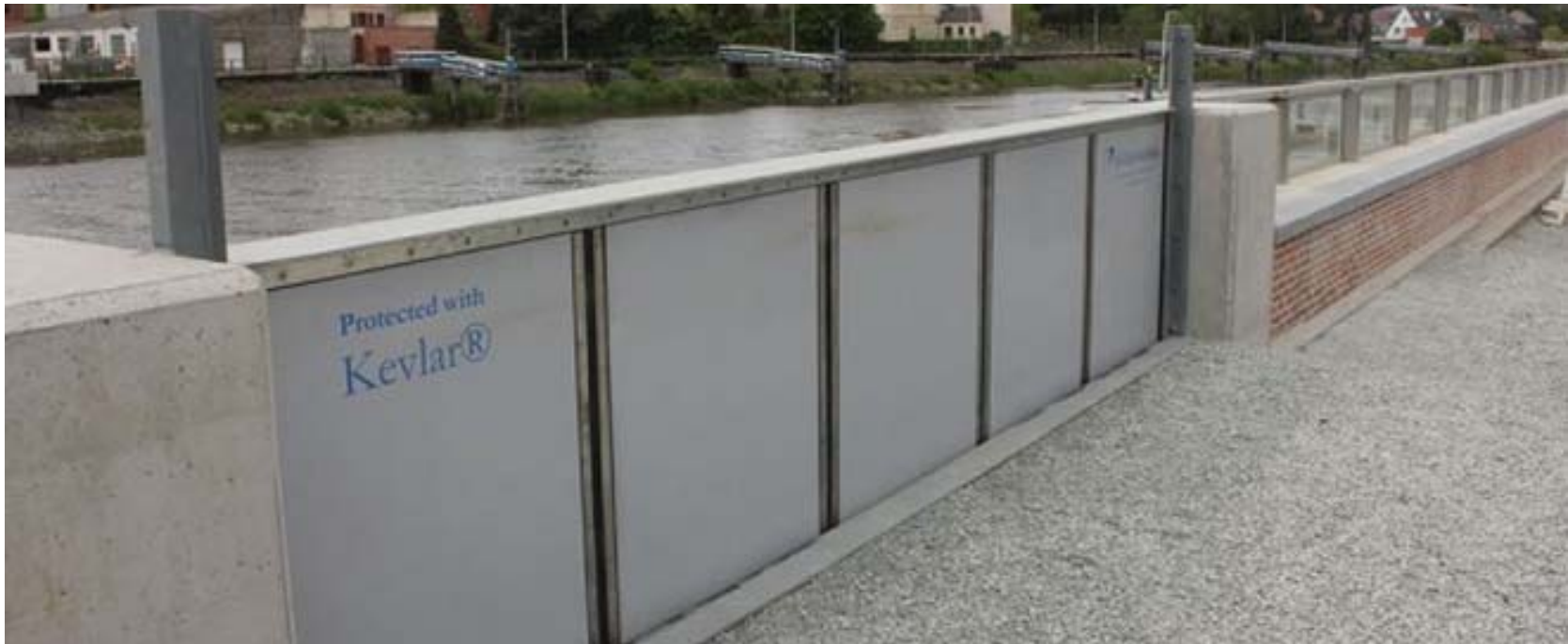
Infill Panel to be Installed to Fill Openings During Storm Events
