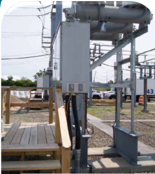
Raise Panels / Equipment
