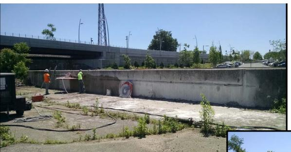
Sawcutting of Existing Floodwall on Trout Brook
