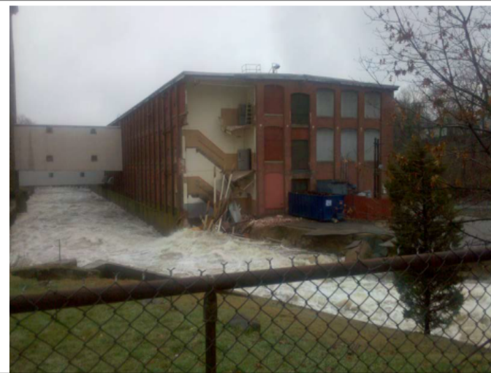
March 2010: Flood flows cause severe erosion of the riverbank. This led to a partial collapse of the Concordia Manufacturing building. As a result, the building was uninhabitable.
