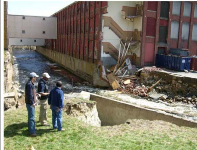
April 2010: Severe erosion has jeopardized the local businesses adjacent to the river, permanent repairs are necessary to ensure employment security and protect critical infrastructure.
