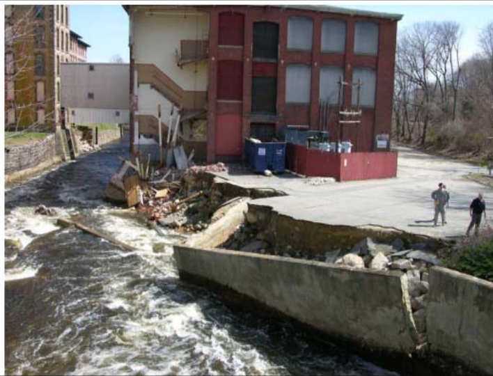
April 2010: Riverbank failure below Laurel Avenue Bridge in Coventry, RI; residents and property downstream need to be protected. The retaining wall collapses into the river.
