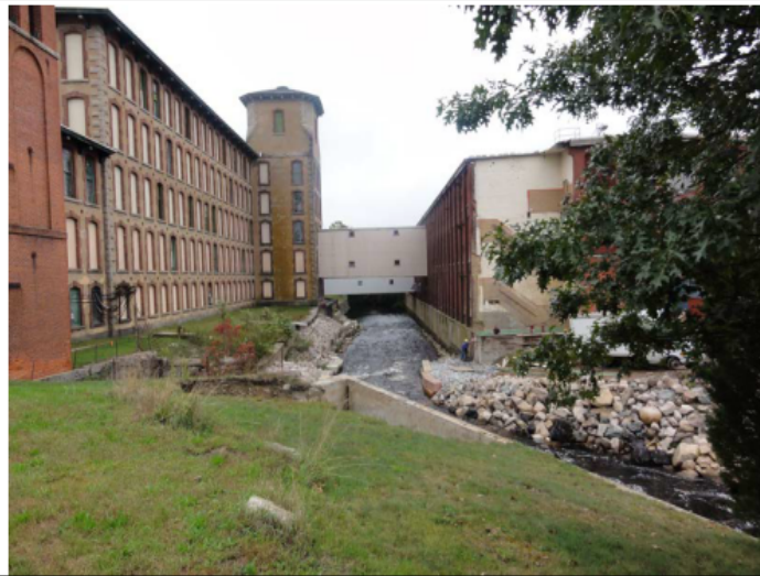
June 2010: NRCS emergency repairs included providing rock rip rap and concrete armor along the toe of the severely eroded riverbank.
