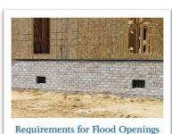
in Foundation Walls and Walls of Enclosures Below Elevated Buildings in Special Flood Hazard Areas In Accordance with the National Flood Insurance Program NFIP Technical Bulletin 1 / March 2020
