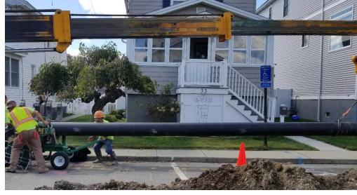
Increased Street Storage and Welded HDPE Installation
