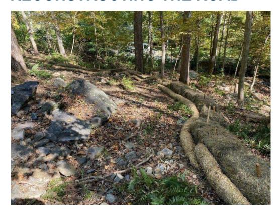
Sediment and erosion controls at toe of slope
