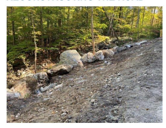
Boulders placed to create toe for riprap armored slope
