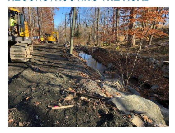
Removal of existing guiderail to facilitate construction
