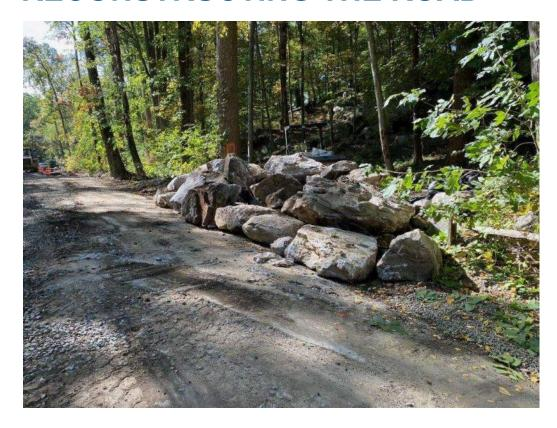
Stockpiled Boulders removed from failed slope to create new toe
