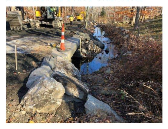
Boulder placement to protect 1930s era culvert
