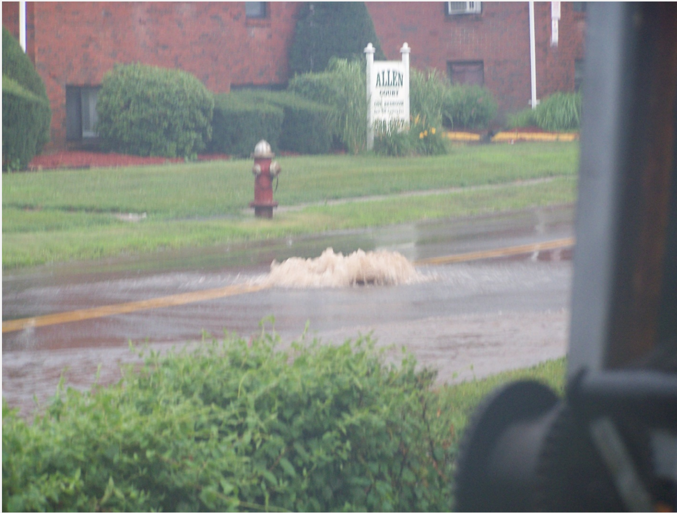
Flooding & Under Capacity Storm and Sanitary Sewers on Allen Street
