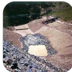
Temporary Sediment Basin
