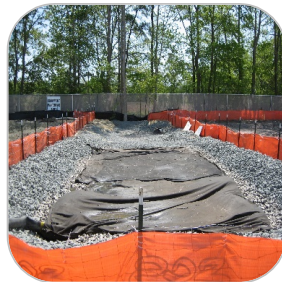
Pumping Settling Basin
