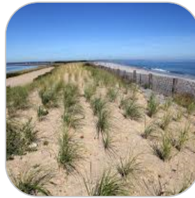
Coastal Bank Protection
