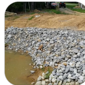
Stone Slope Protection
