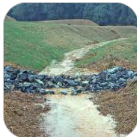
Stone Check Dam
