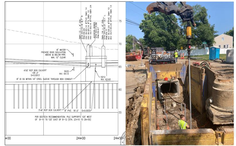
Piles were used due to the poor soils in the area
