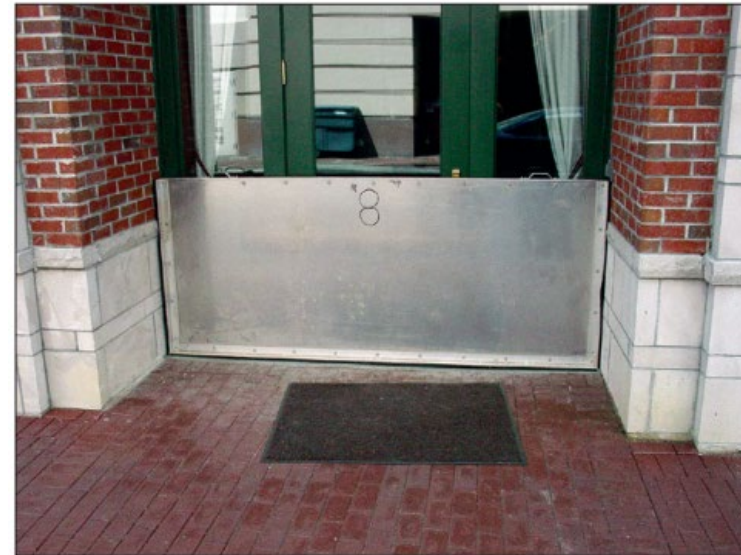
Figure 3-9. Aluminum flood shield used for flooding less than 3 feet deep
