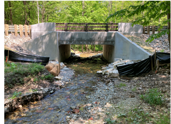
Replacement of undersized and perched culvert
