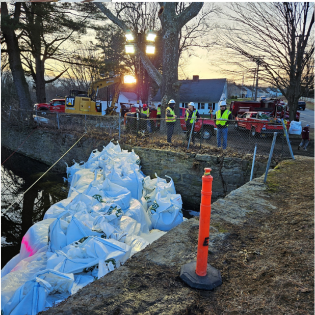
Emergency Placement of Cofferdam at Fitchville Pond Dam, Bozrah, CT
